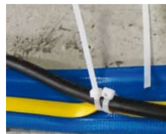
Secure Power Cable to Hose
